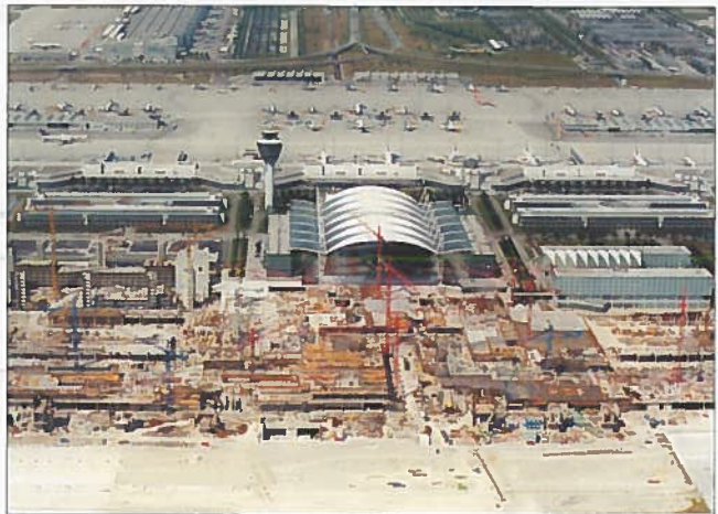
The new Terminal 2 under construction at Munich Airport. Copyright Werner Hennies/FMG
